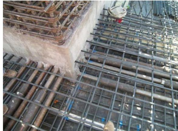
(a) Collector connection to shear wall boundary zone
