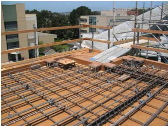
Figure 9-3 – Confinement of a collector.
