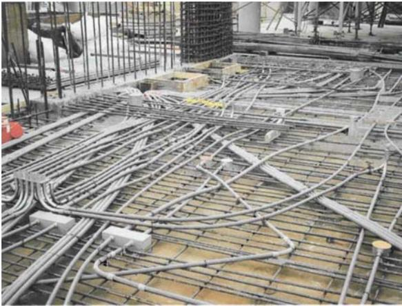
**Figure 9-5** – Embedded conduit.
