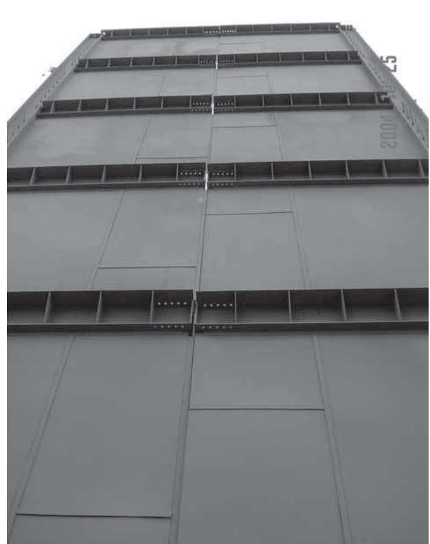
Fig. 1–32. Close-up view of wall at mid-span splice location, ING building (courtesy of Louis Crepeau and Jean-Benoit Ducharme, Groupe Teknika, Montreal, Canada).
