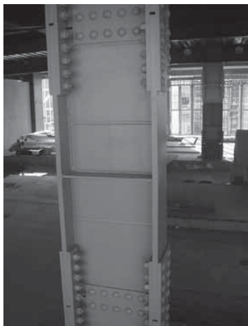
Fig. 1-4. Intermediate column approach used in Japan (courtesy of Takanaka).
