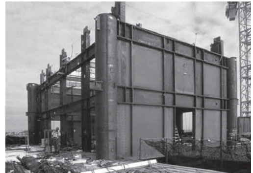
Fig. 1-20. Core walls with composite concrete infill steel pipe columns (Seilie and Hooper, 2005).
