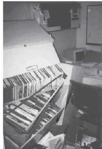
Fig. 1-15. Nonstructural damage in Olive View Hospital due to 1994 Northridge earthquake (Naeim and Lobo, 1997).
