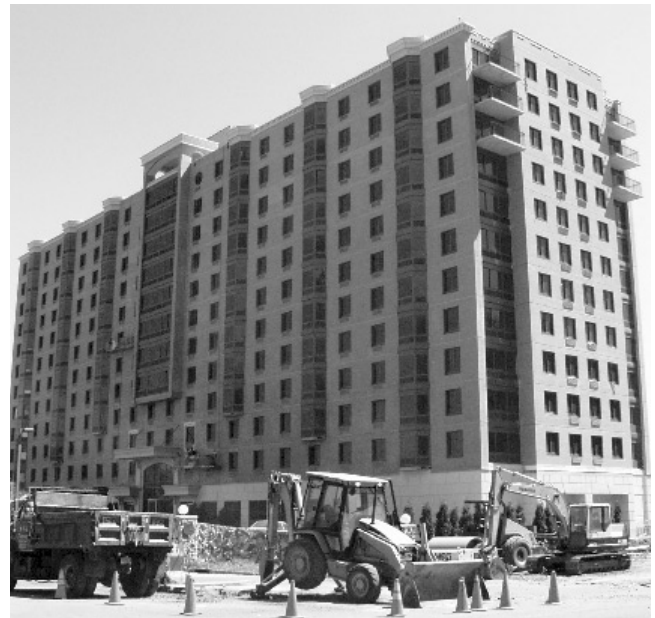
Fig. 1.3 Staggered truss apartment building.
