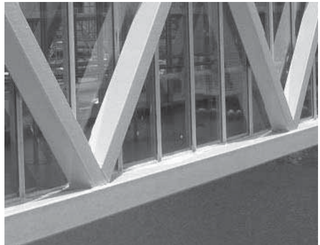
Fig. 2-1. Stepped HSS-to-HSS connections.
